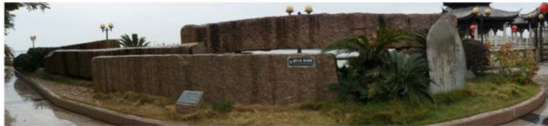
Figure 1: Ancient granite stone beams of the Guangji bridge (number 12), preserved in a park near the bridge. The spans range between 10 and 14 m.
